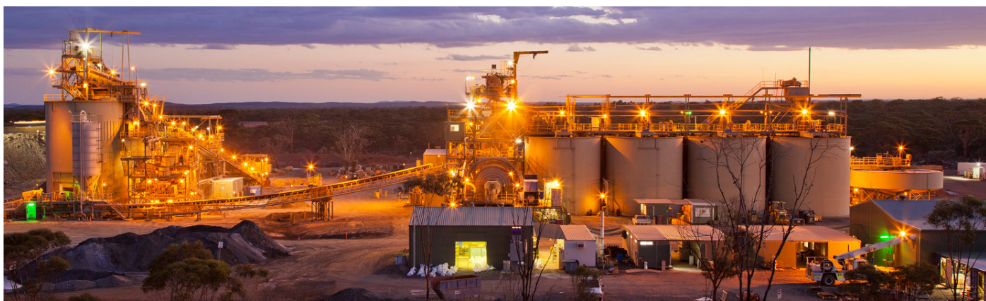
[Picture: Higginsville Gold Plant 1.35 Mtpa]
